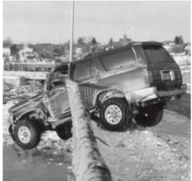
An accident on the Carlton Bridge in Wiscasset. Mainers pay more than $1 billion a year in costs associated with inadequate, unsafe highways and bridges.
